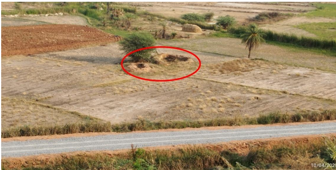
Figure 2.5 Sand boils on downstream side
