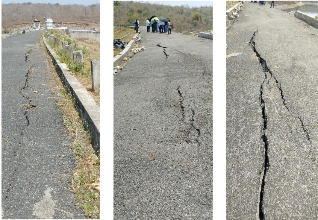
Figure 2.2 Cracking in earthen dam
