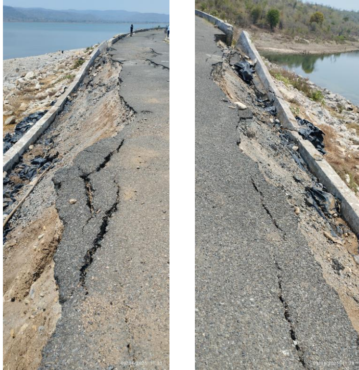
Figure 2.3 Slides in earthen dam
