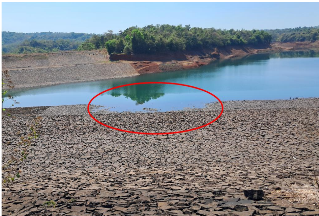
Figure 2.4 Indication of upstream berm settlement
