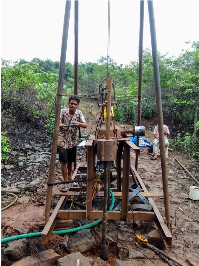
Figure 3.1 Rotary drilling at dam site
