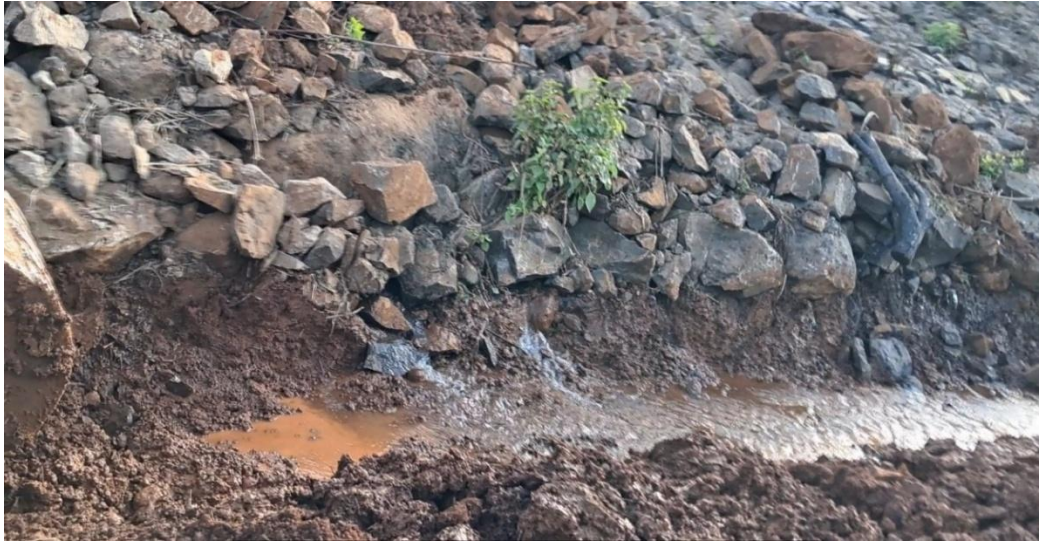
Figure 4.1 Excessive seepage on downstream berm of earthen dam
