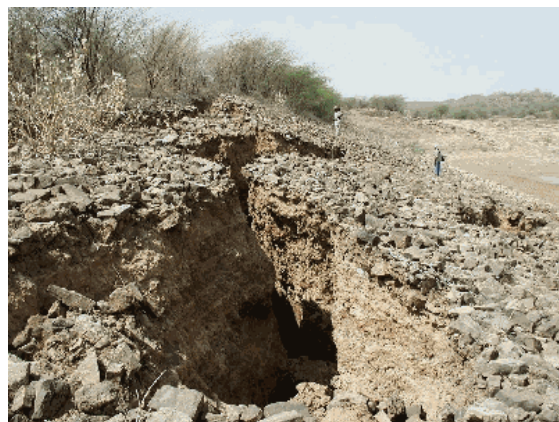
Figure 6.2 Cracking at Shivilakha dam, Gujarat
