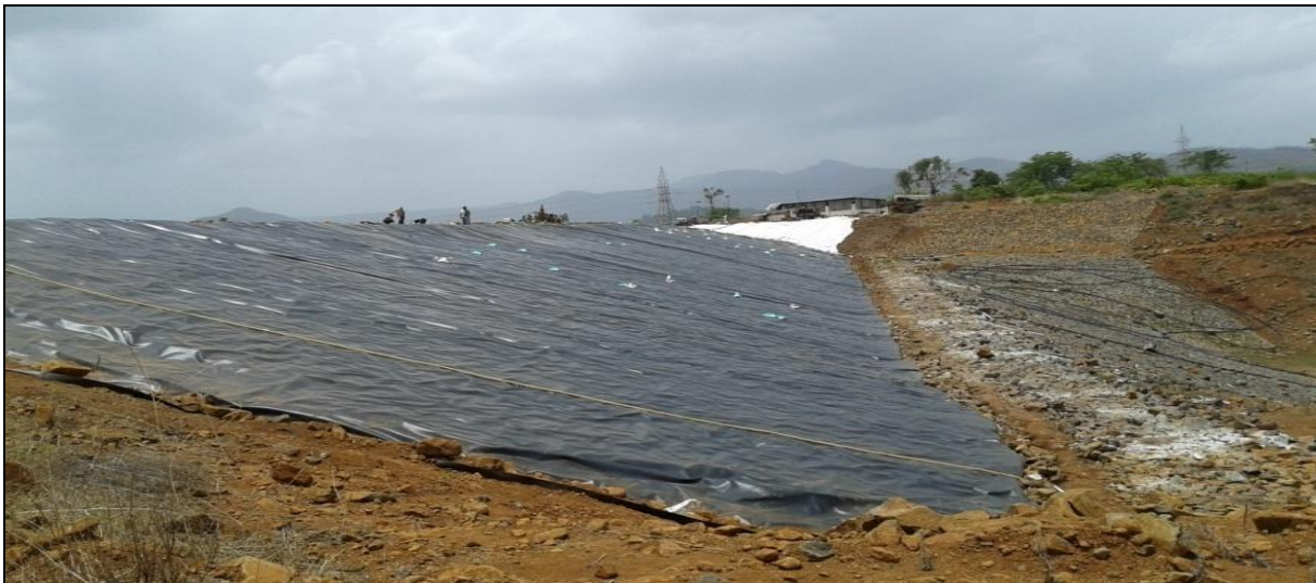
Figure 9.8 Installation of geomembrane on upstream face
