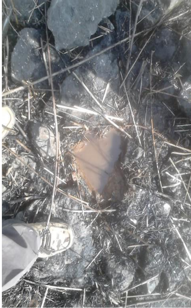
Figure 4.7 Seepage water accumulated on top berm at EL 130.5 m
