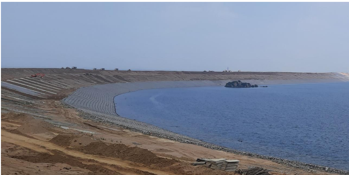
Figure 7.4 Installation of stone pitching for upstream slope protection
