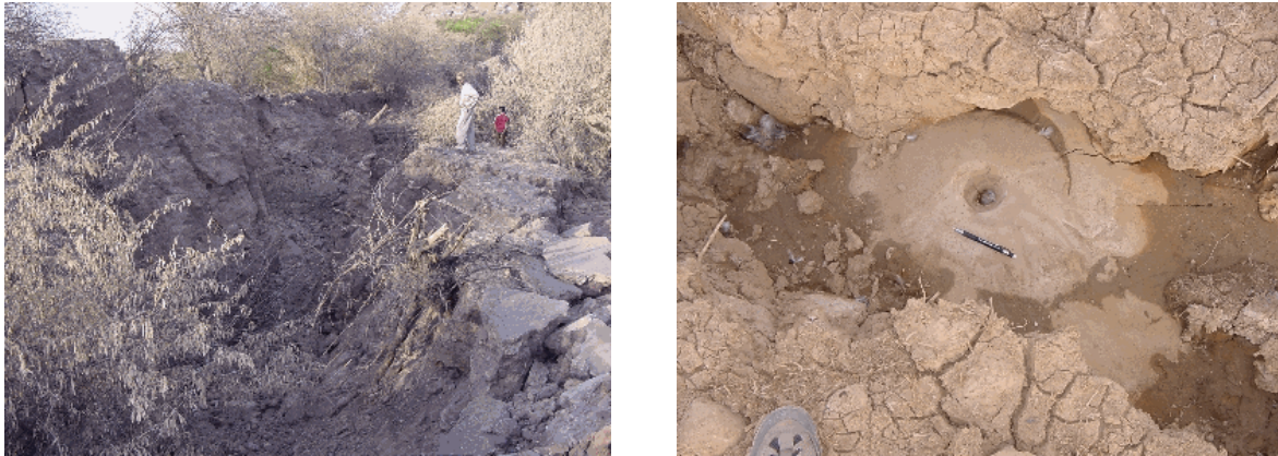
Figure 6.3 Widespread liquefaction, cracks and sand boils at Chang dam, Gujarat
