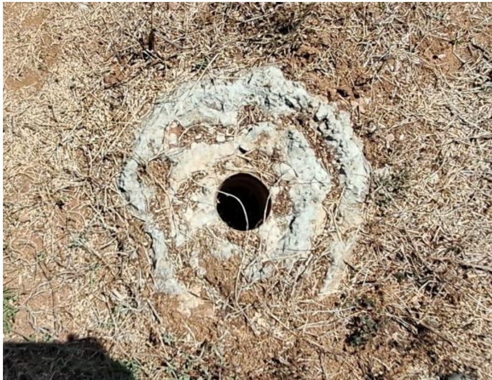
Figure 7.2 Grout holes for grouting through dam body
