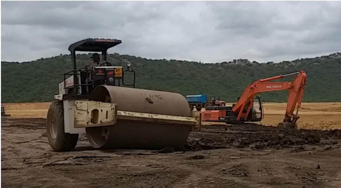
Figure 7.3 Soil Compaction
