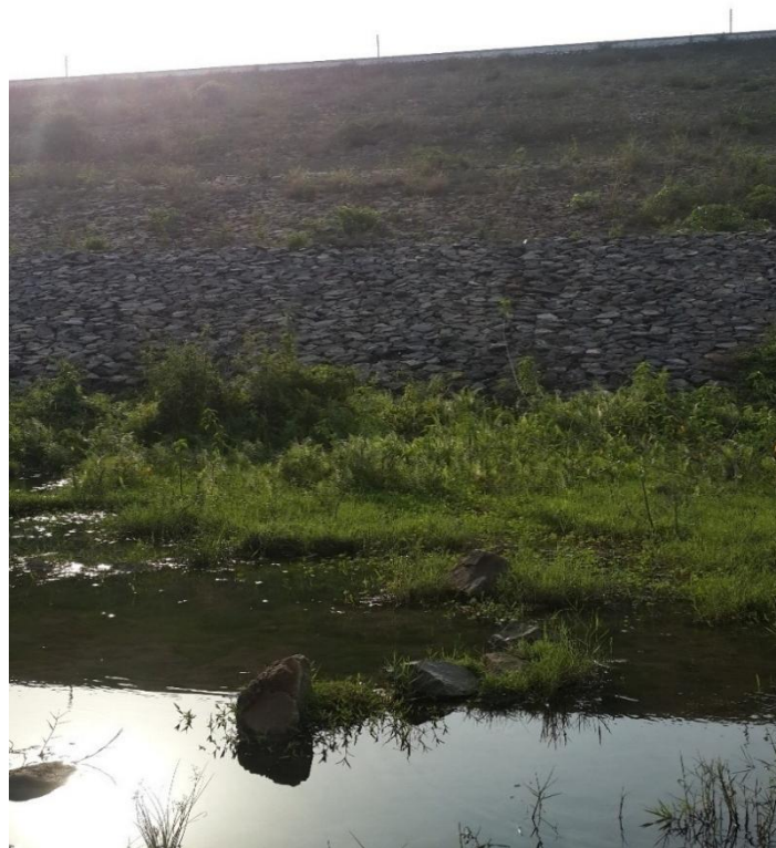
Figure 4.2 Seepage near downstream toe of earthen dam
