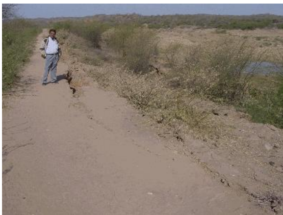
Figure 6.2 Cracking at Shivilakha dam, Gujarat
